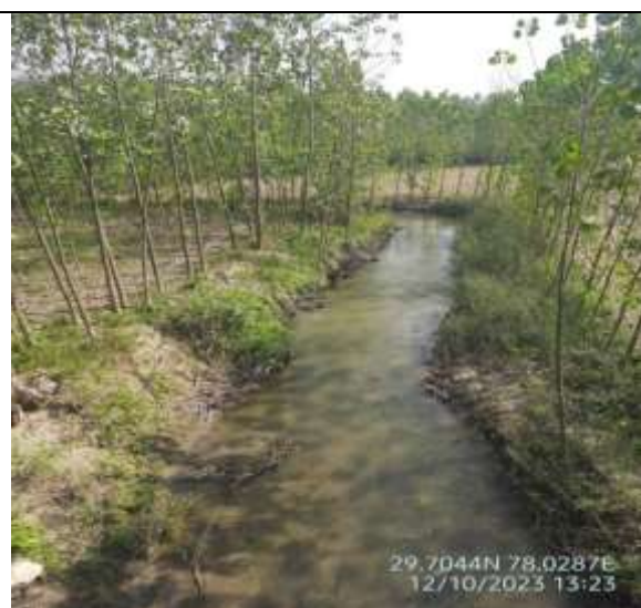
Figure 32: Hadwa drain before confluence with Laksar drain
