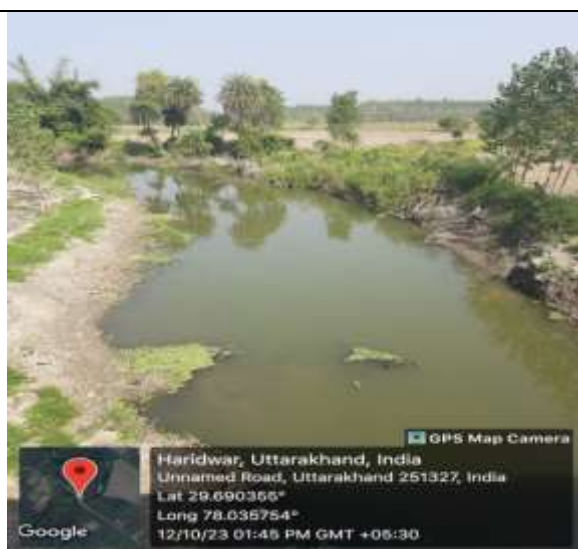
Figure 33: Laksar drain after confluence with Hadwa drain
