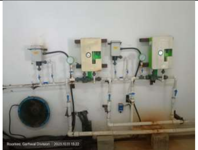
Fig 6: Gas chlorinator
