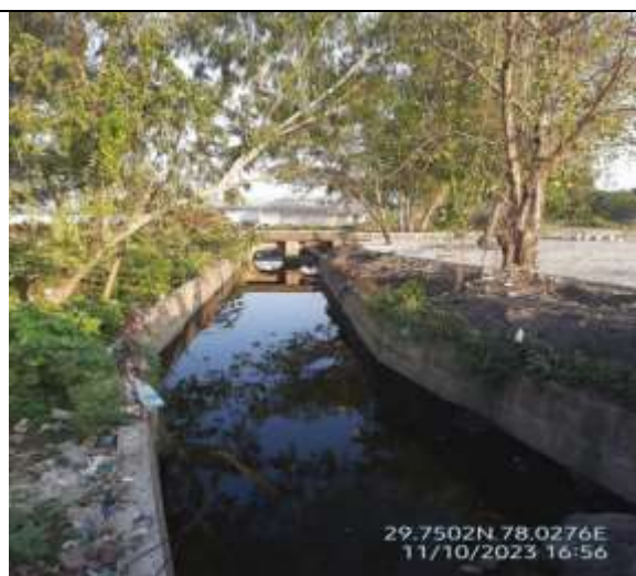
Figure 28: Laksar drain upstream of unit
